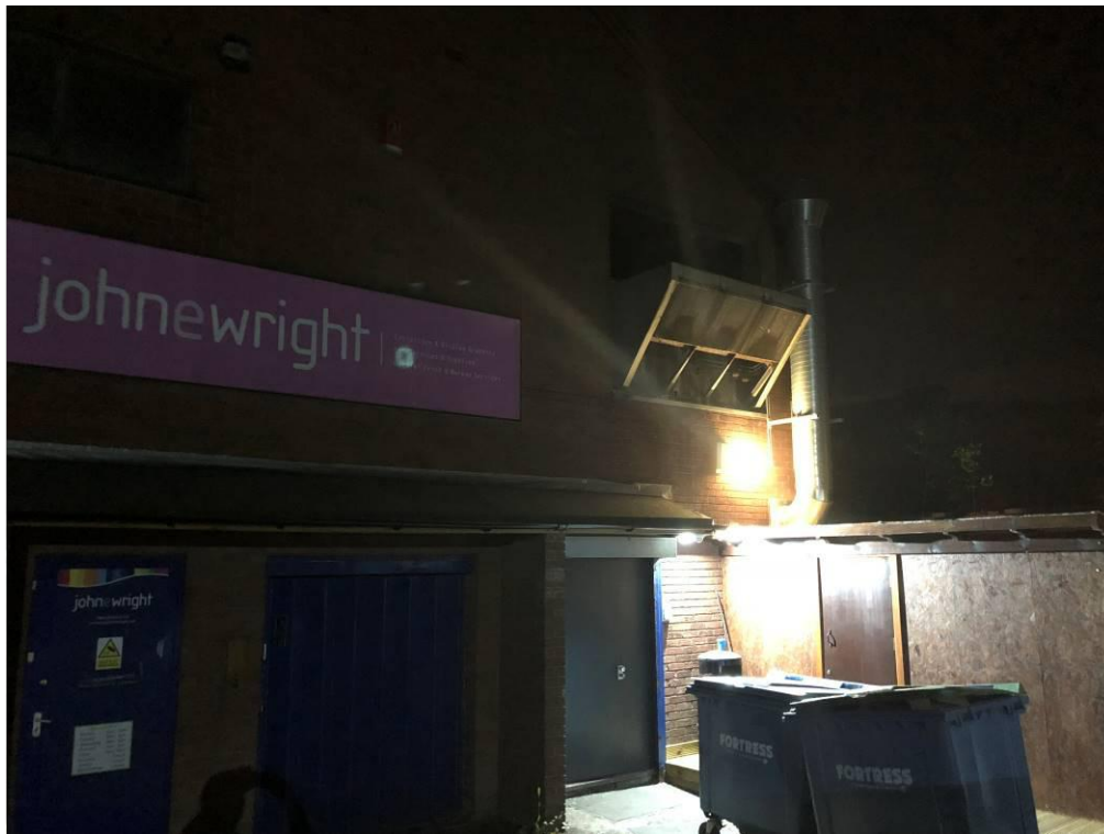
Plate 1 – View showing kitchen extract to rear of Tiki Hut.
